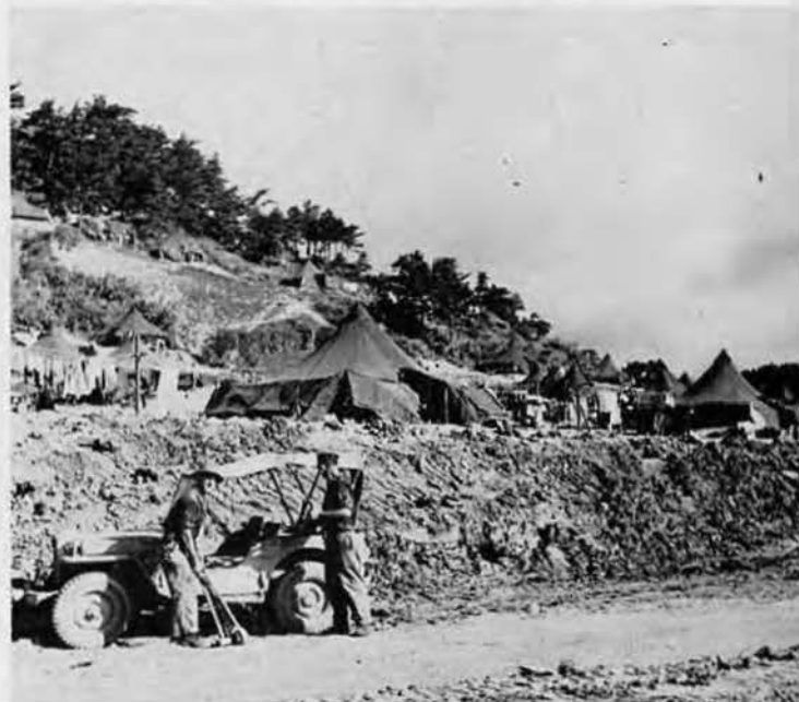
Roads and spots for the tents were gouged from the slope
