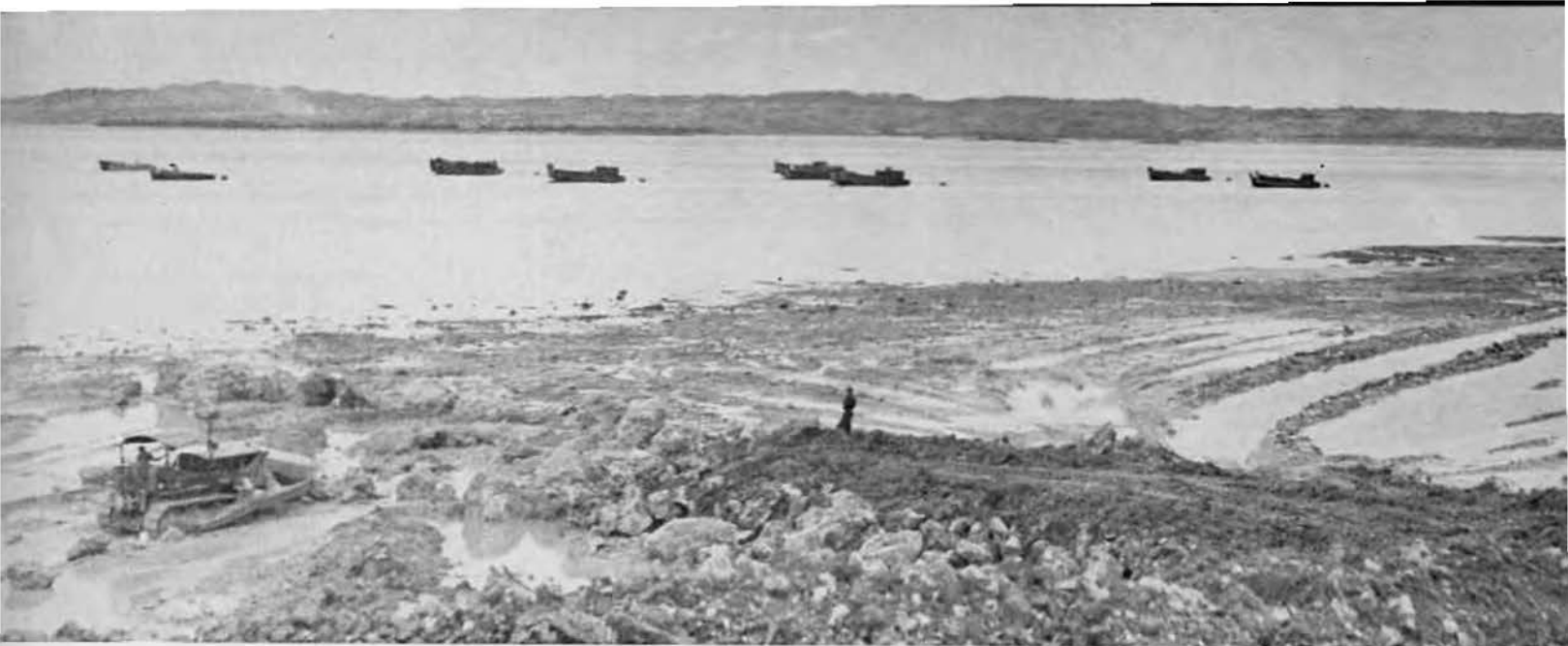
Fill material gradually formed an approach for the Section Base pier.
