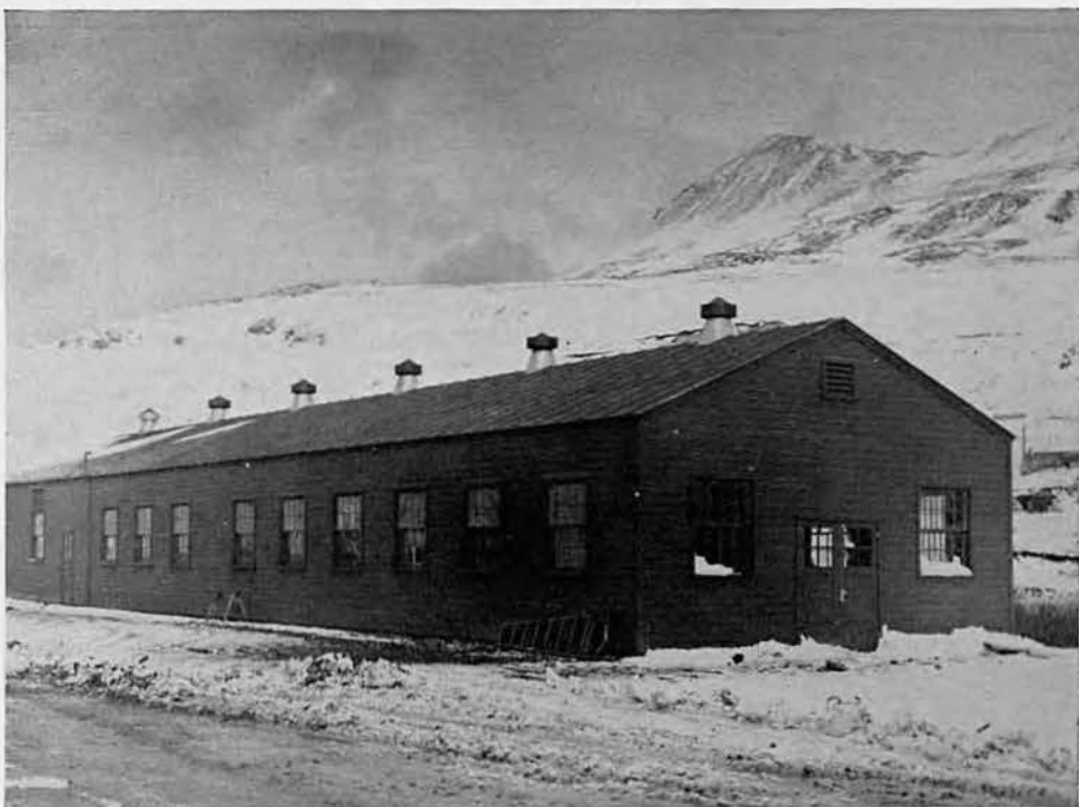
In slush and under dark, wet skies, we built much around Dutch Harbor. This warehouse is a small sample.
