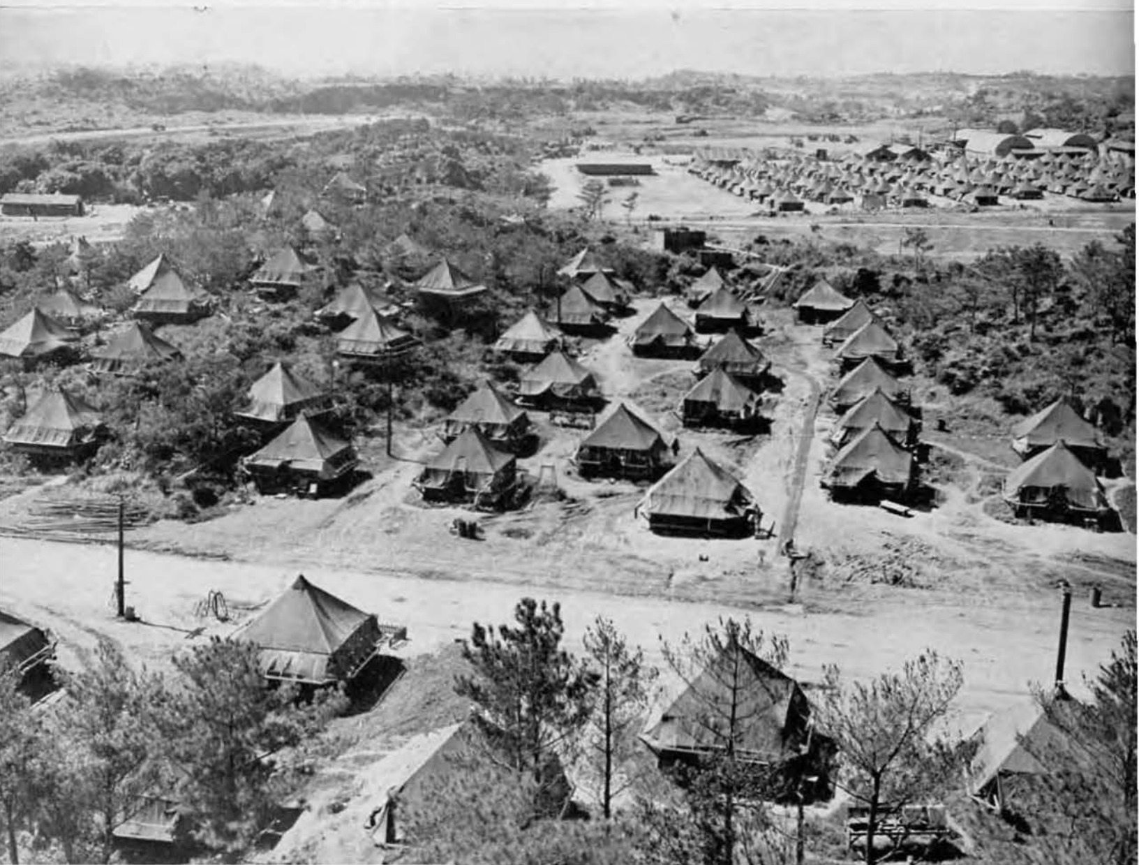
Looking west, tents covered the knolls as well as the flat spots. Beyond, the 86th battalion pitched orderly tent rows. The CNCT (Commander Naval Construction Troops) camp was in quonset huts in the right distance.
