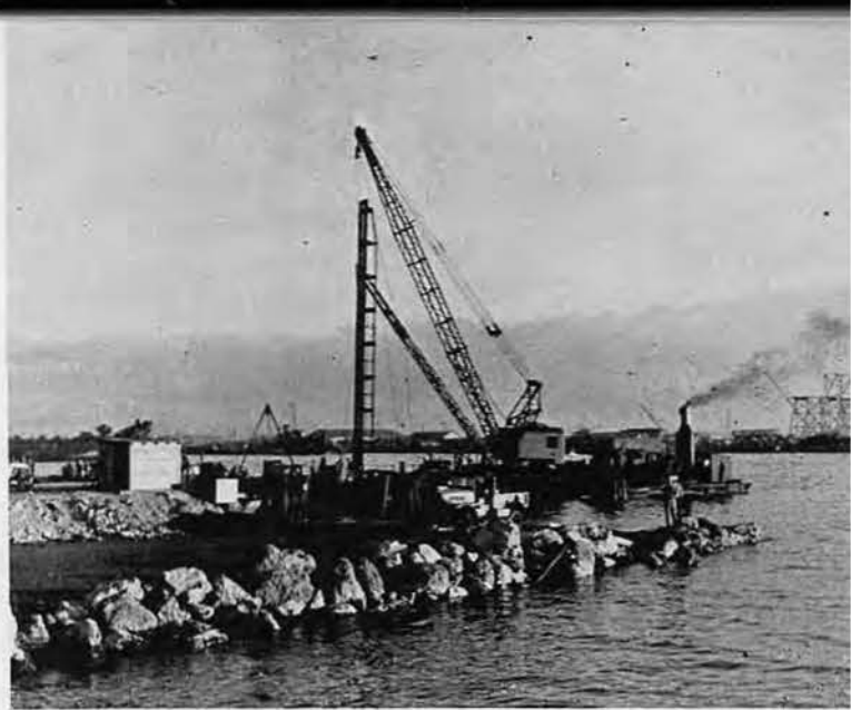
A BARGE SLIP was built at Iroquois Point to handle airplane-loaded barges. Aircraft were stored on a large field in this area. The slip helped to speed the transfer of the planes from ships to the field and from the field to the carriers.
