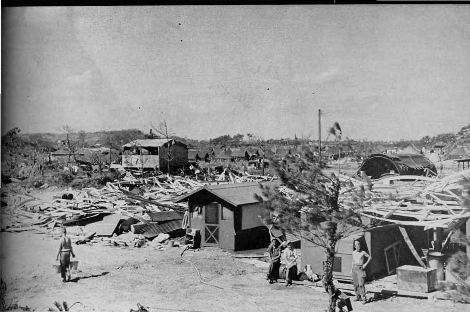
The pieces of the galley and mess hall—two large quonset huts—were peeled off like a head of lettuce; then the huts collapsed
