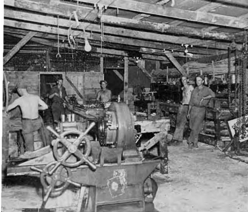
The Plumbing Shop put in lots of pipes
