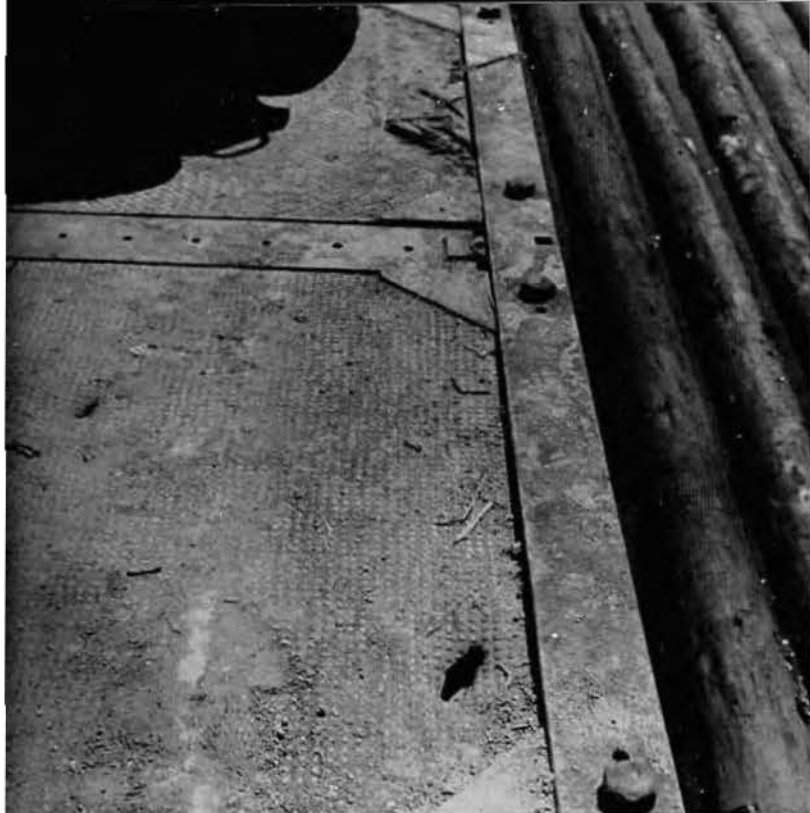
Shrapnel from a Jap bomb punctured pontoon cells on May 17
