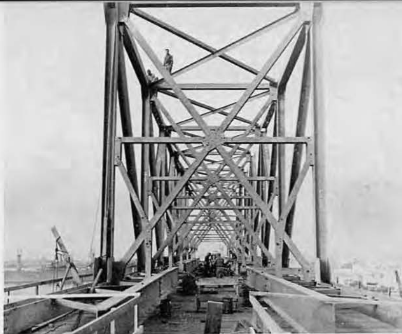
The top of the steel was 90 feet in the air
