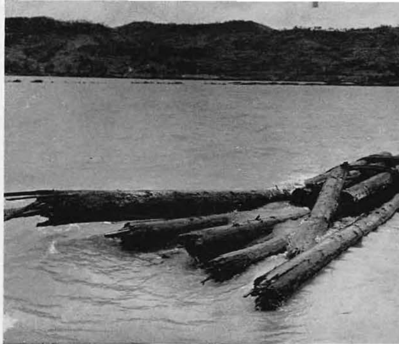
When an LST rammed the pier, it sheared off a dolphin
