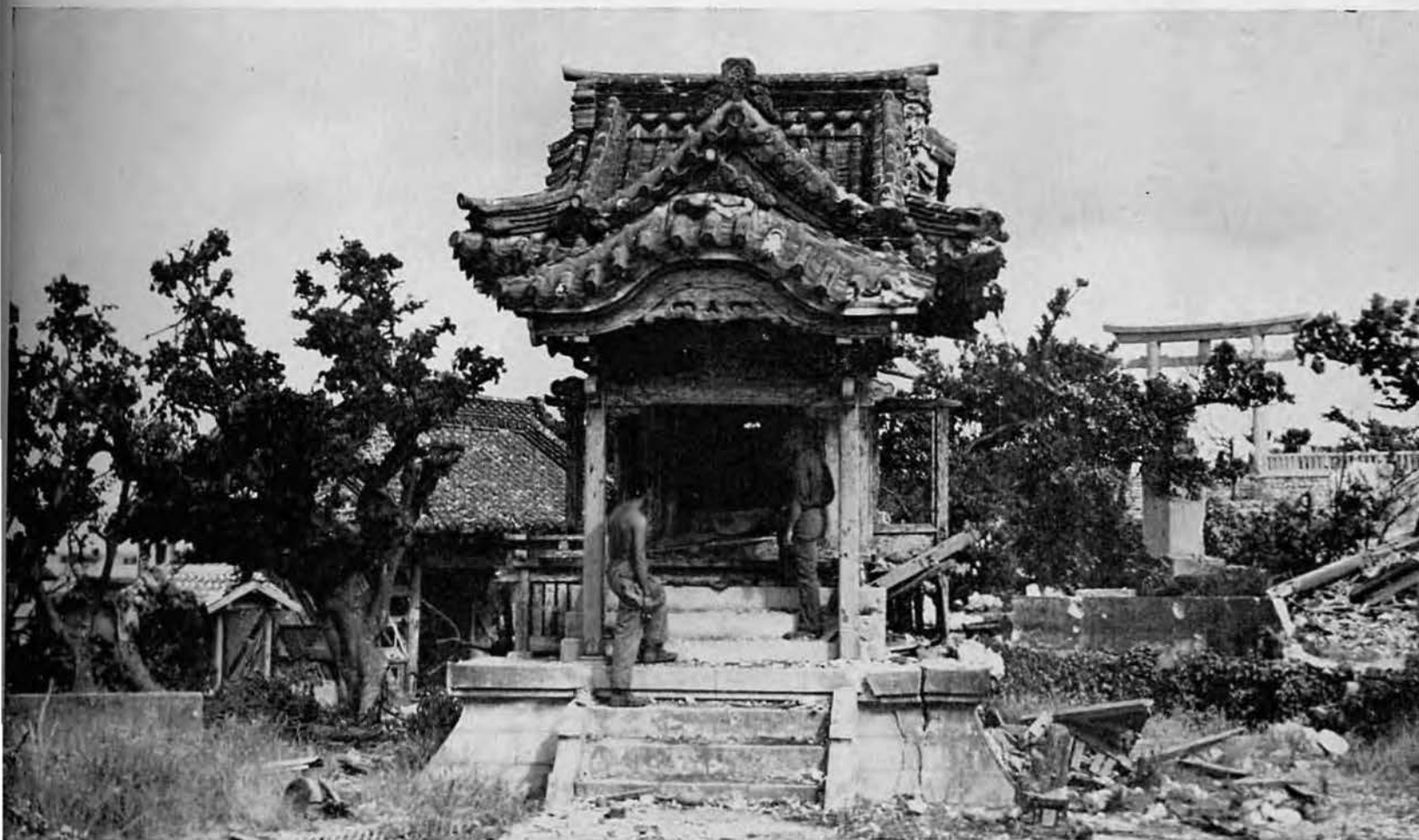
Top: Sandbags had not been much protection
