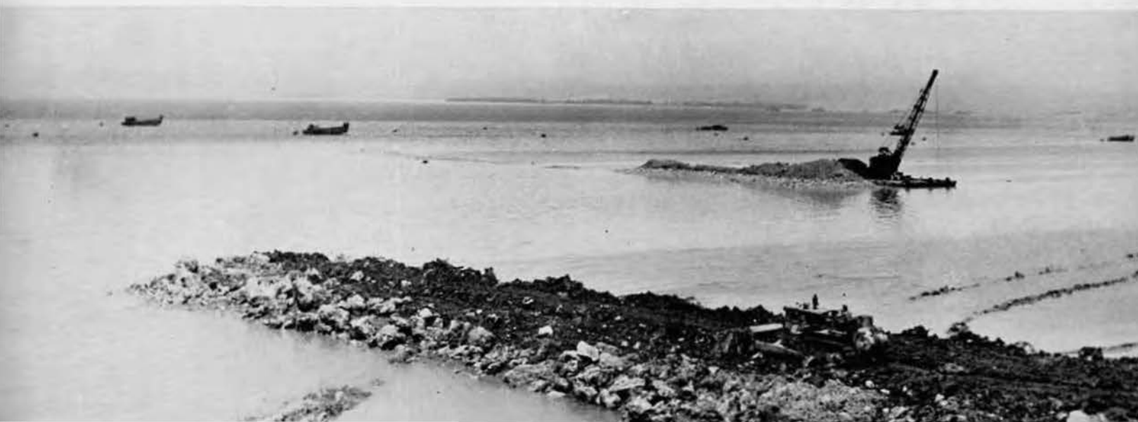
Below: The pier approach moved out into the bay.
