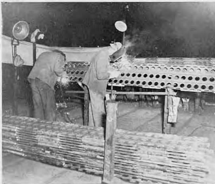
Hinge pipes were welded to each mat section
