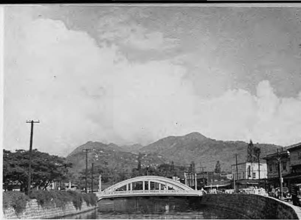
Honolulu climbed up the hills from the canal and River Street
