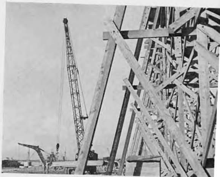
Heavy, bolted timbers formed the trestle
