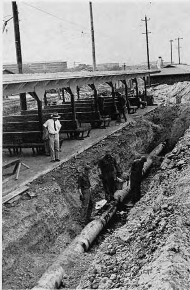
A BERTHING FOR FUEL BARGES was developed near Halawa stream. Old moorings were removed; nineteen dolphins were driven; a timber catwalk was built; pipe lines were laid; a machine shop, office, galley, and living quarters were erected. Soon Navy Yard oilers were using the berthing to supply the ships.
