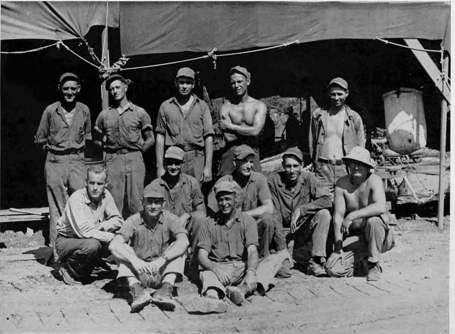
Top: When mud was deep and water rushing, Welders Kirkpatrick, Ricks and Witter turned out thousands of feet of drainage pipe made from 105-mm. howitzer shell cases.
