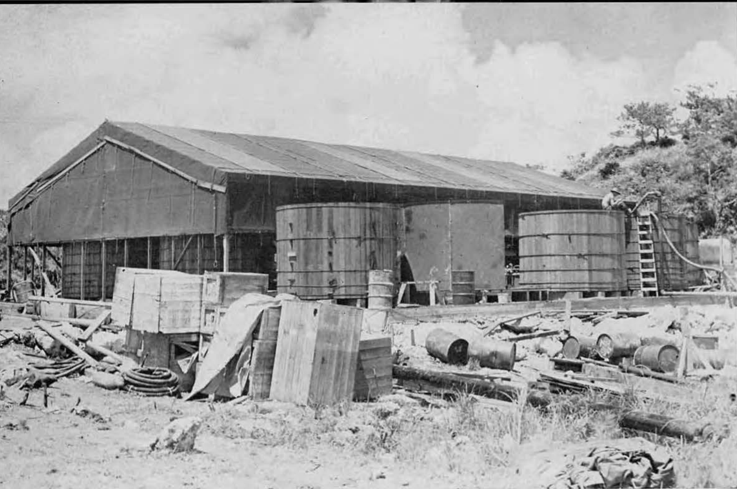
Clear, clean drinking water was made at the rate of 160 gallons per minute by our water works
