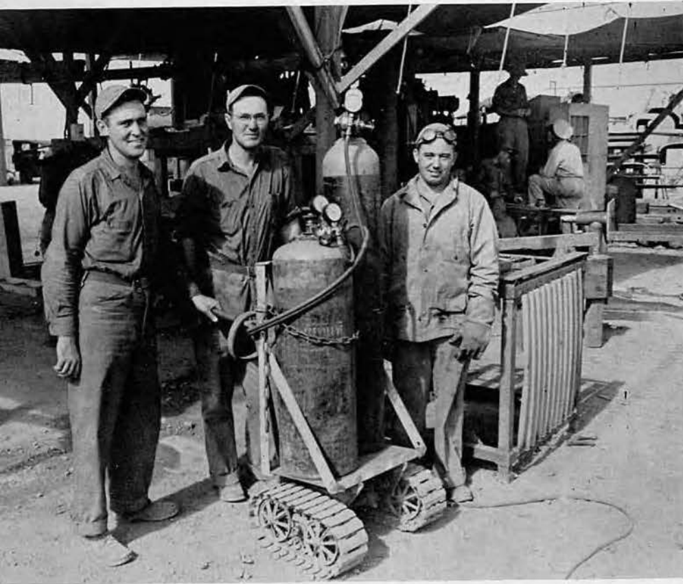
Seidenberg, Wyatt and Garrison put junkyard caterpillar rollers from an old bomb carrier on to a field welding tank so that it could be pushed easily over the roughest terrain.
