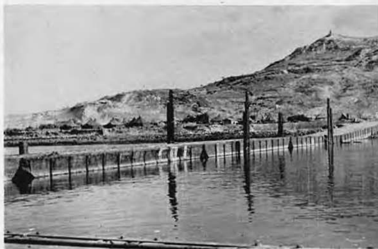
The right-hand approach to the Yonabaru pier was used first by LST's on July 3.
