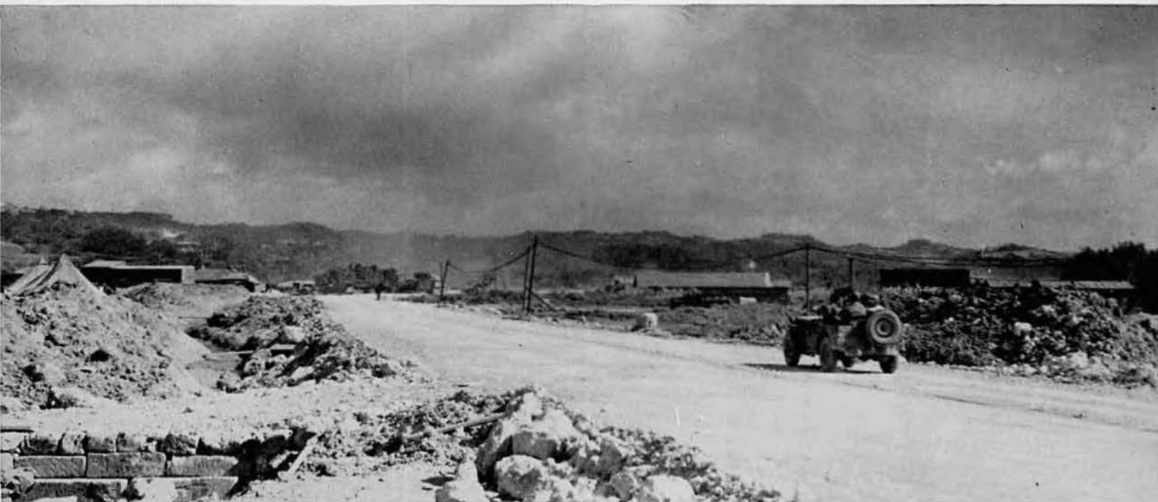
Top: A bulldozer and dragline filled in the last section of Highway 13 on which Blackjacks worked Bottom: When the weather dried up a little, Highway 13 had a solid coral base and surface
