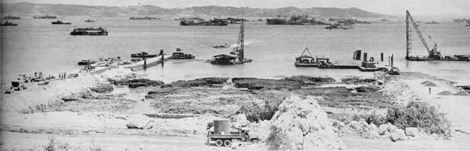
The approaches neared completion
