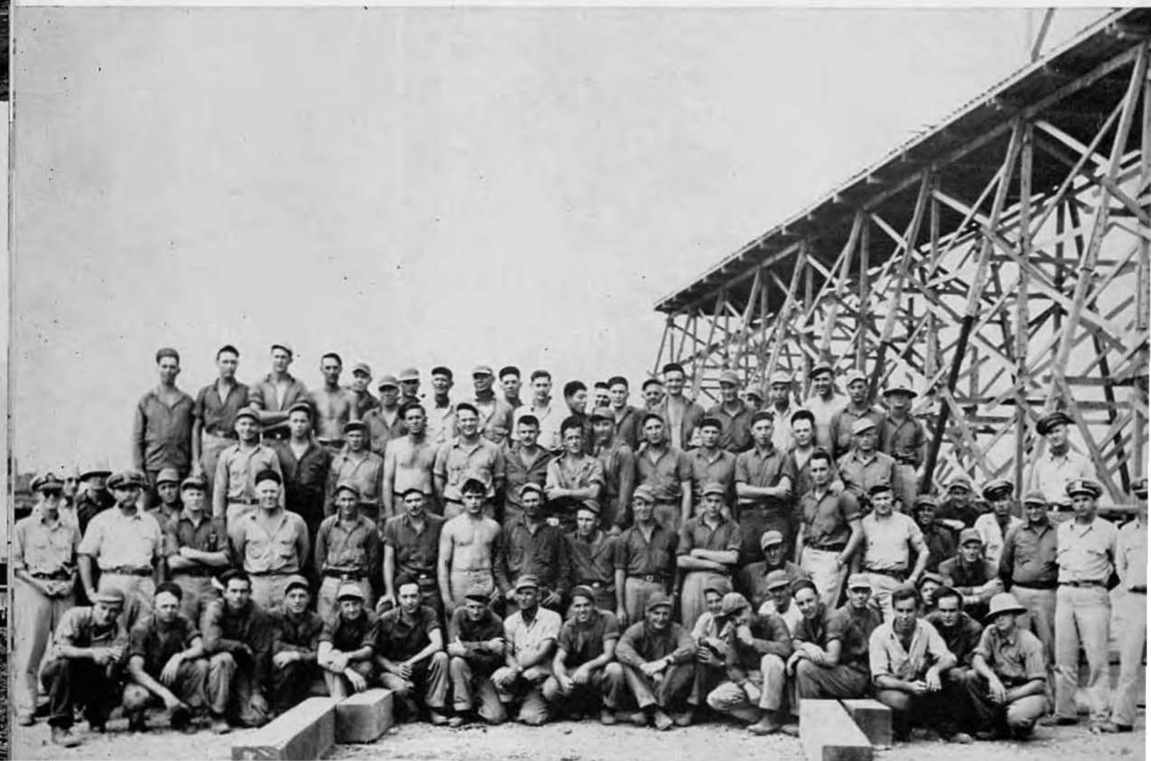
The gantry crane crew were rightly proud of their accomplishments
