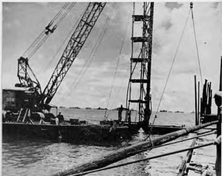
Available piling was spliced into 100-foot lengths for the deep water.
