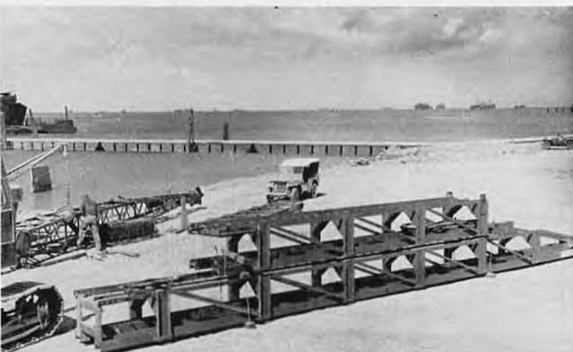
A needed pile driver was improvised from a crane
