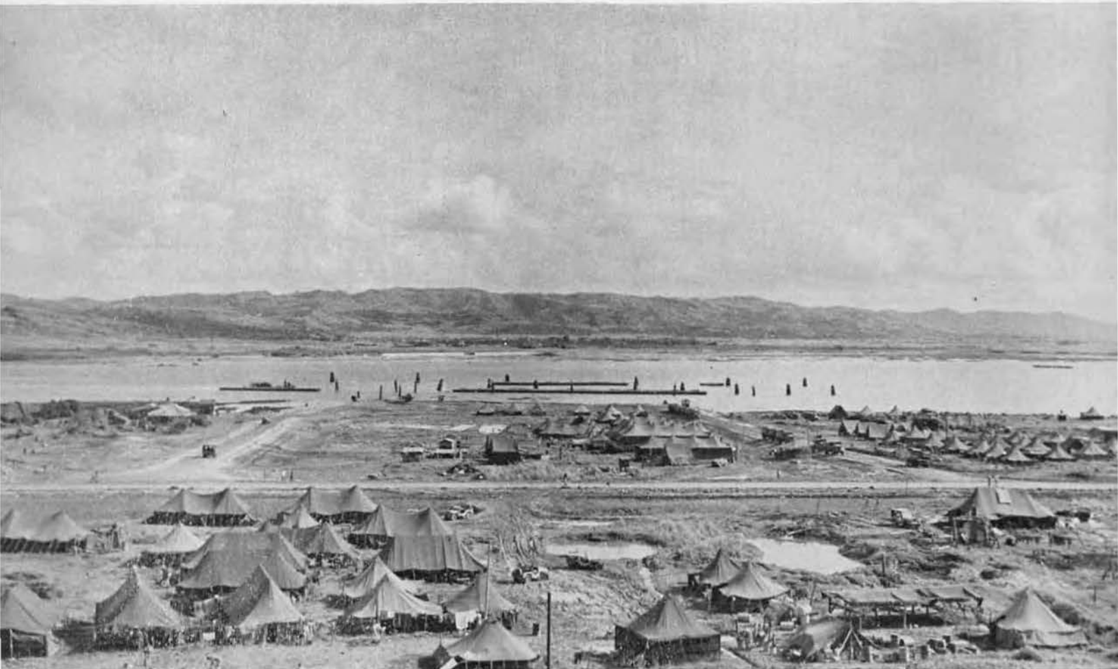
Top: Eleven LST's used the pier at one time. Though its life was brief, the Yonabaru pier paid off Bottom: The hard storms of the last of July and the first of August destroyed the Yonabaru pier
