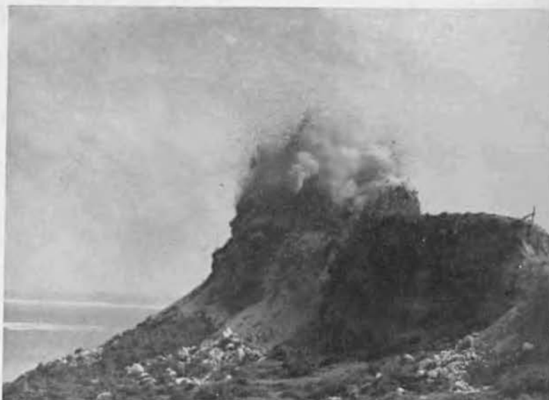
Many 300-hole charges were blasted in the quarry near China village.
