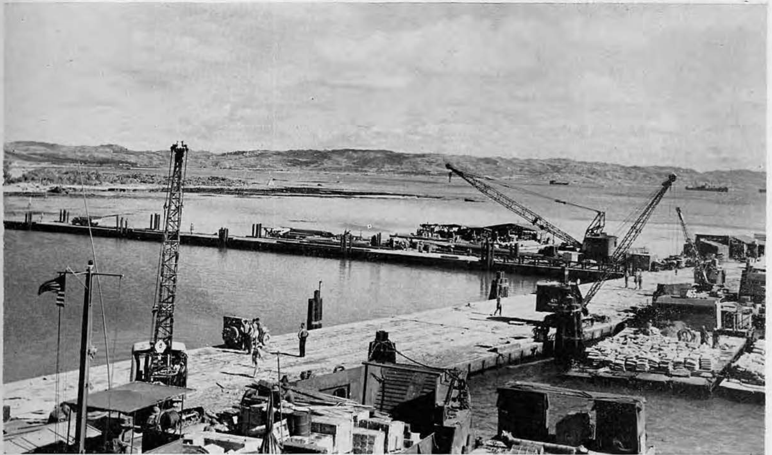
Later, as the Naval Operating Base began to move to Baten Ko, the pier's length was extended and a second approach was put in.
