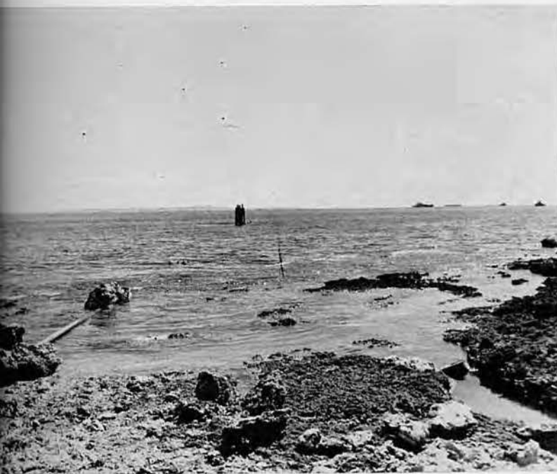
Dolphins were driven for sea-loading tanks
