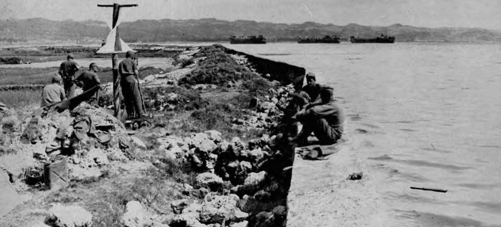
Our surveyors laid lines for our first pontoon pier while our LST's were still on the tidal flats
