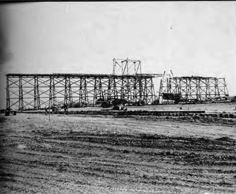
The first steel began to rise on January 5
