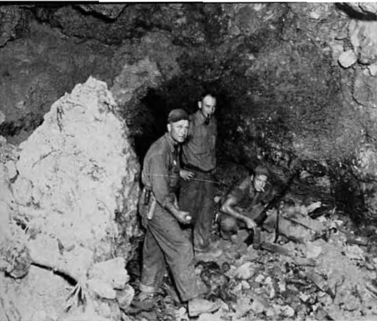
Goodman, Odenius and Dykes inspected a cave after the Jap ordnance had been exploded.
