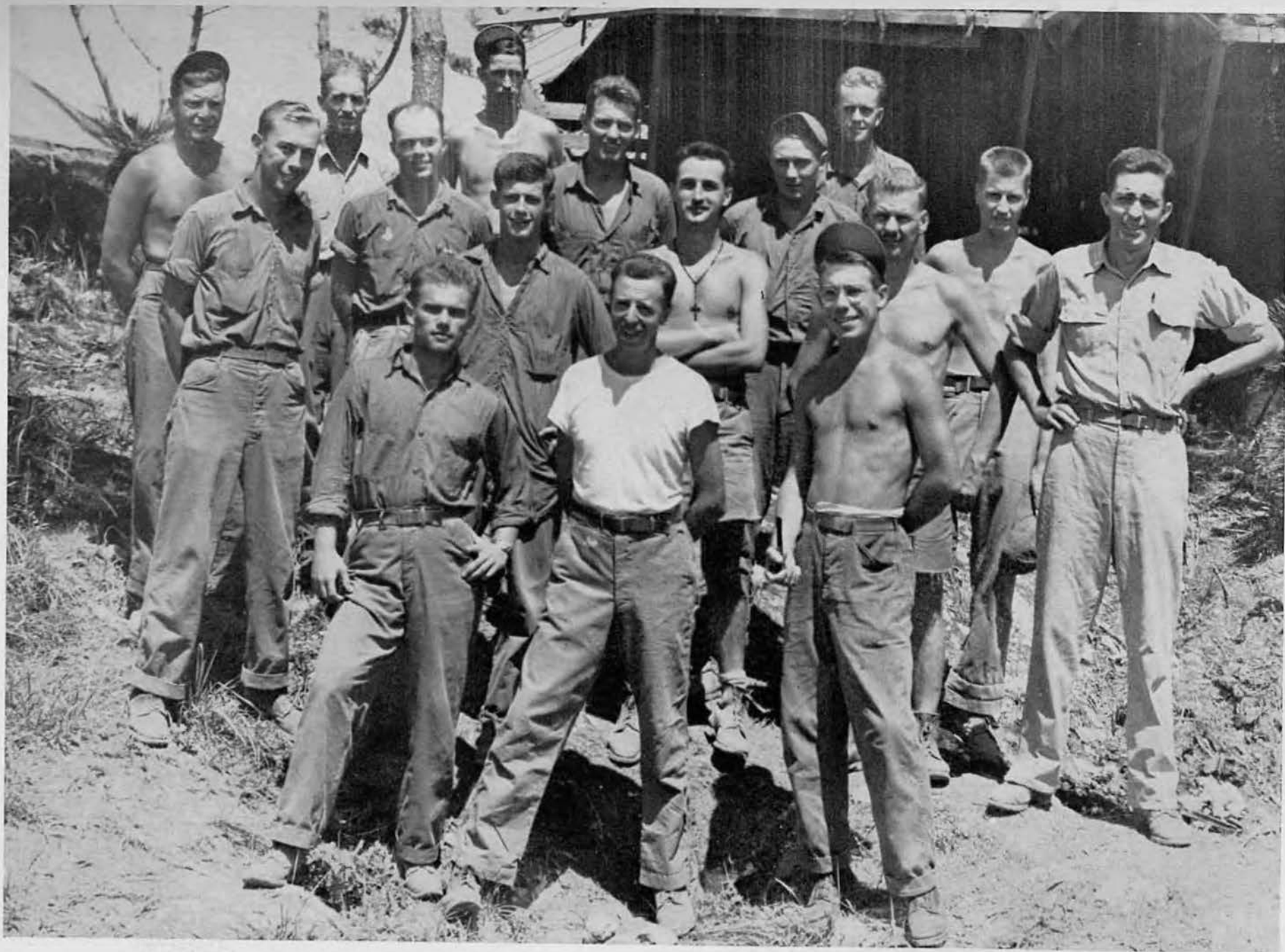
The surveyors and draftsmen of the Engineering Department did the groundwork for every project. Surveying while the fighting was still on had its dangers. Rule O. Seymour received a Purple Heart for wounds received when a booby-trapped grenade blew up when he tripped it while surveying.
