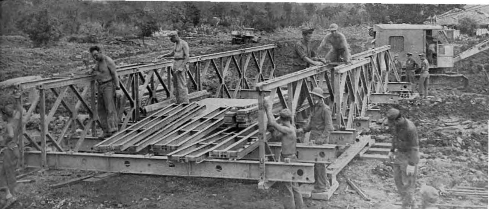
Seabees adopted the Bailey bridge for some low spots and put them together as fast as the more experienced Army engineers.
