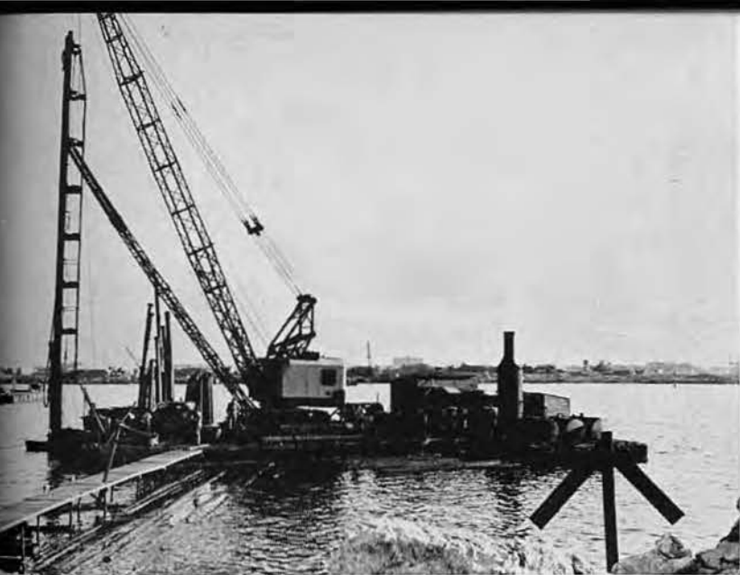
A BARGE SLIP was built at Iroquois Point to handle airplane-loaded barges. Aircraft were stored on a large field in this area. The slip helped to speed the transfer of the planes from ships to the field and from the field to the carriers.
