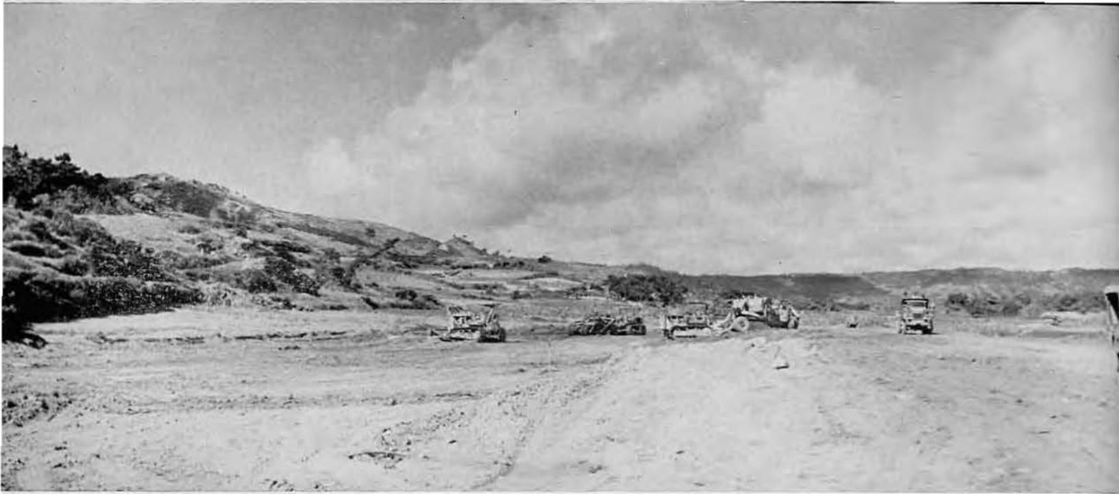
Heavy equipment widened the old Jap road along the south shore of Buckner Bay
